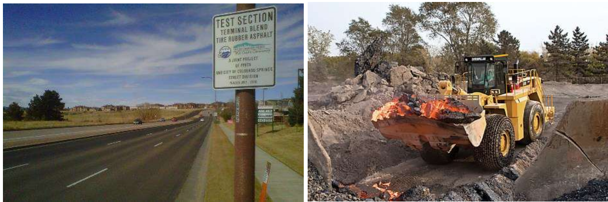
Figure 1.6-12.: photo of asphalt treated draining base made with EAF slag in Colorado Springs, 2010 [4], and photo of Moving 1200°F hot slag to a cooler pile in Charleston, SC with a 988H Wheel Loader
