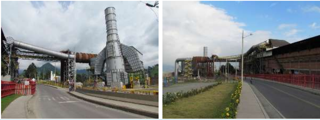
Figure 1.6-11.: photo of an existing baghouse of similar size of the one which will be adopted by PURE FONTE LTÉE, currently installed in a plant of the Ternium group (photo by Tenova)
