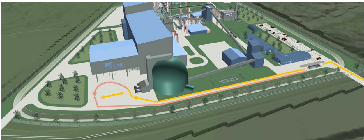
Figure 7.2-2.: 3D representation of the IO pellets arrival and unloading into the dome.
