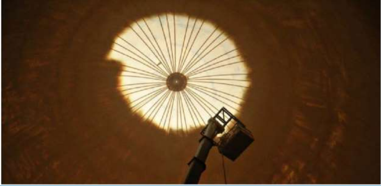
Figure 10.3-3.: Primer applied in advance of polyurethane insulation [1]
