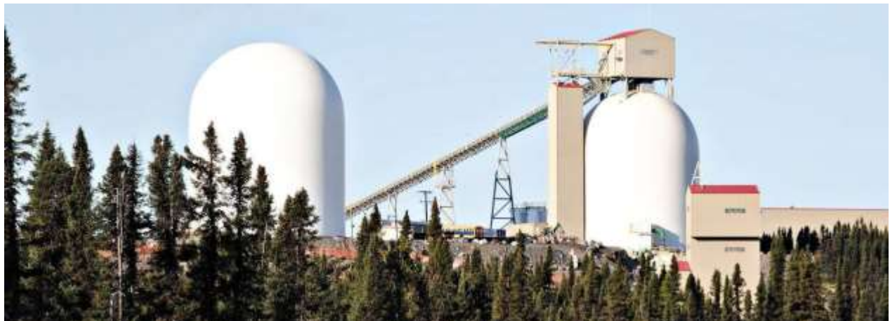
Figure 10.3-2.: IO bulk storage dome silos constructed by Dome Technology in Fermont, Québec [1]
