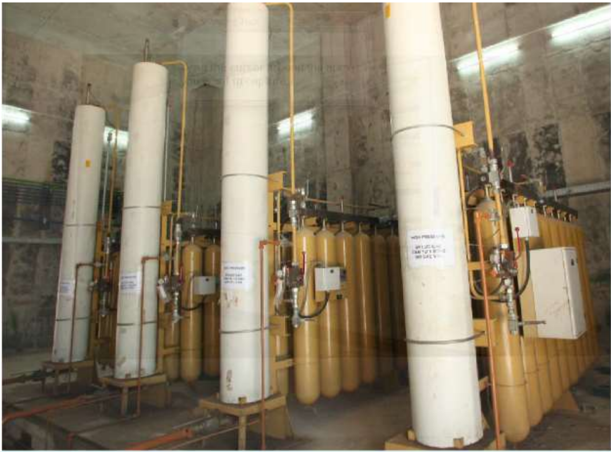
Figure 10.3-44.: Typical Hydraulic Accumulators
