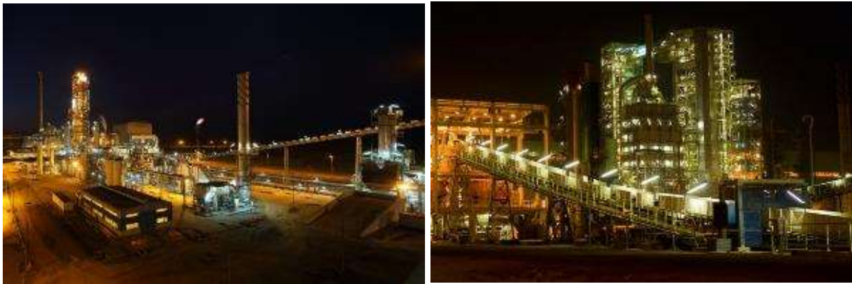
Figure 1.5-2.: Energiron® DRI plant at Ezz Steel, Egypt [3]
